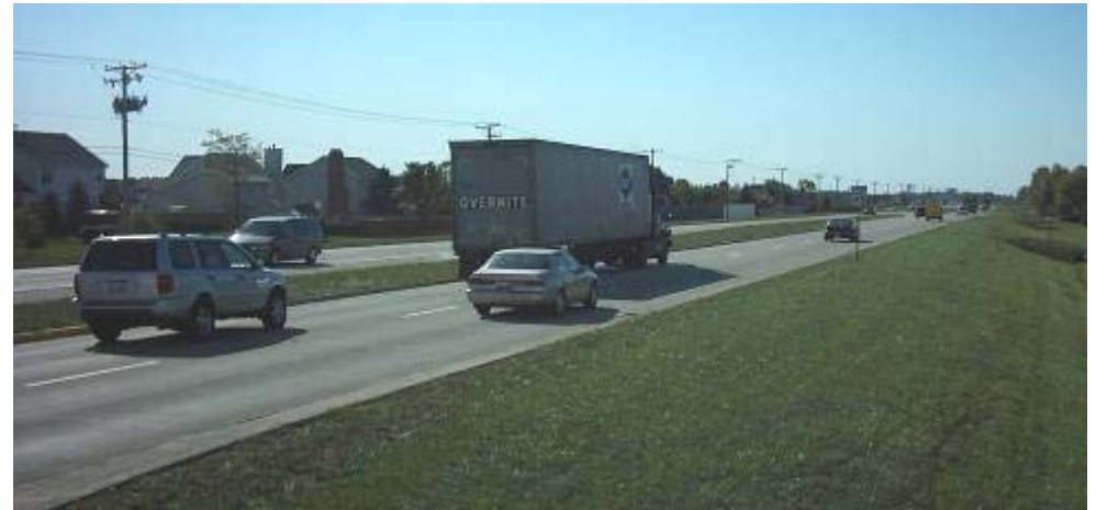
IL 59 southbound in southwestern Naperville/northern Plainfield
